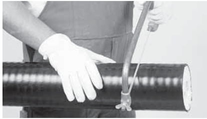
2 Cut the casing pipe with saw.
