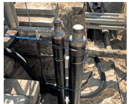
Proper securing and fastening of the connections
