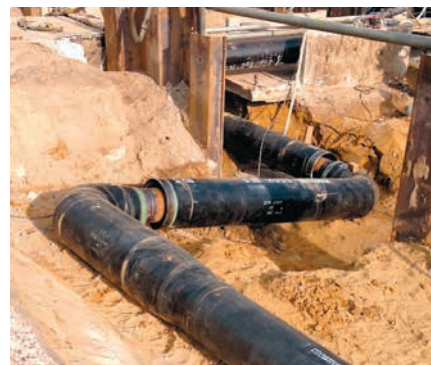
BRUGG-STAMANT® Safety Pipe with expansion element
